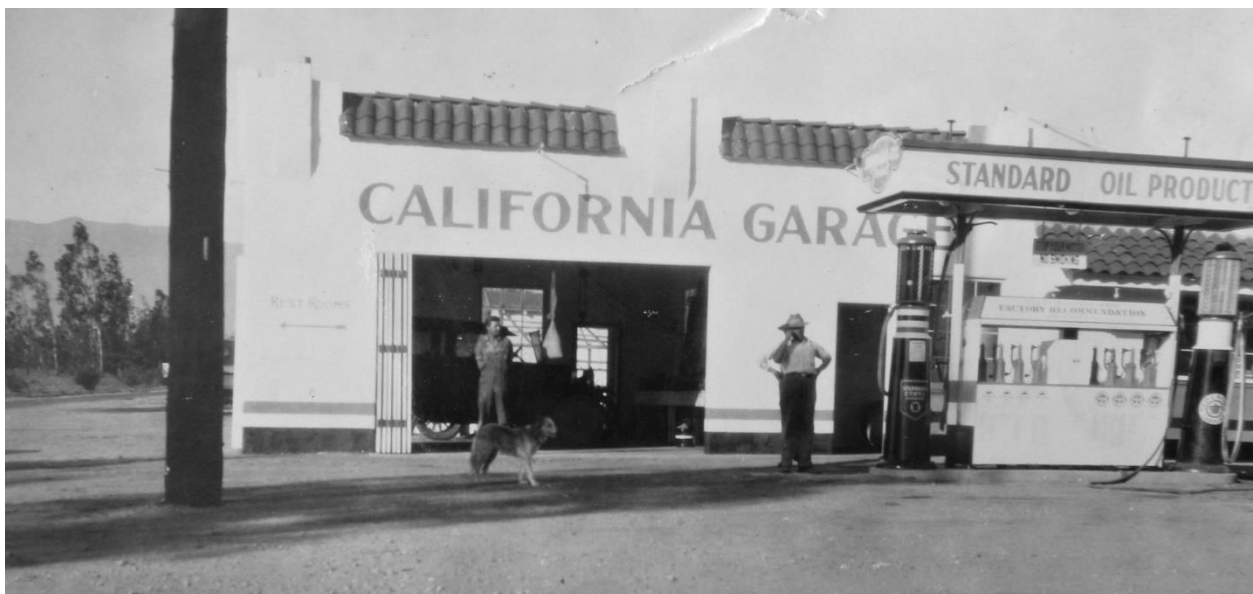
California Garage in about 1929 on U.S. Route 70/99 (13930 Valley Boulevard in year 2020)
