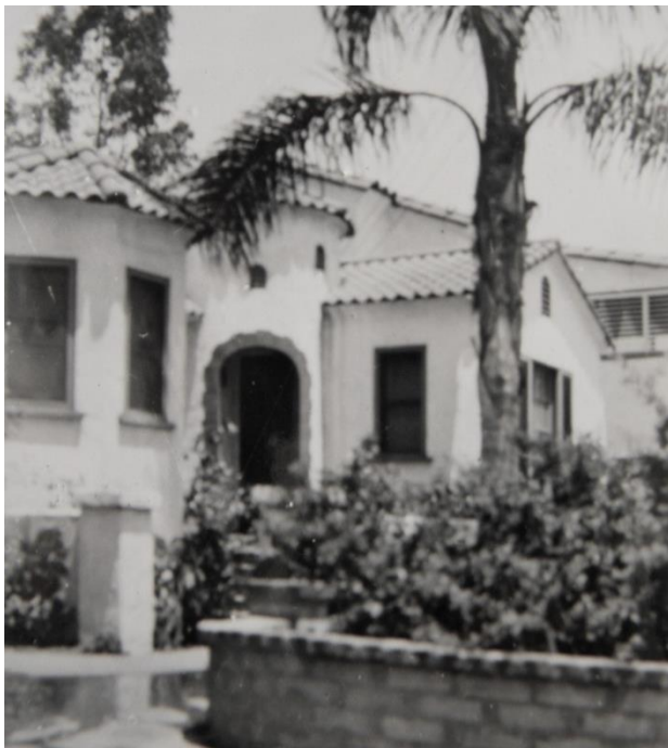
The Segna home after the new addition.
